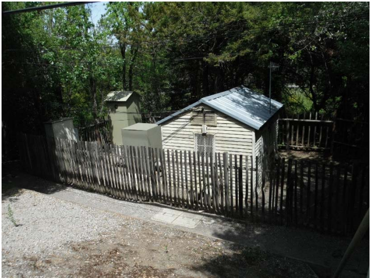
View from Portola Road
